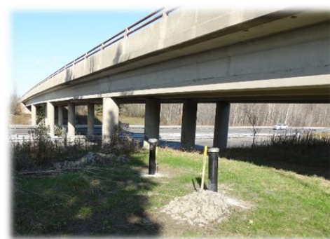
Photo 1: Fraser Road Underpass
